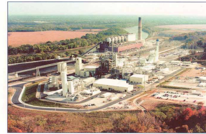
The Wabash River Coal Gasification Repowering Project
